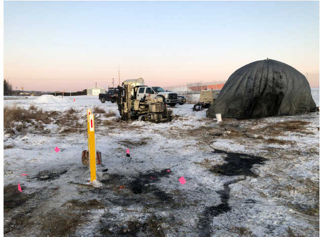
Photo 8: PlumeStop injection November 4, 2019
