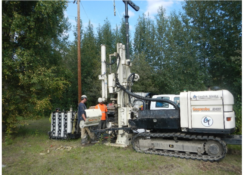
Exhibit 2-1: Monitoring well installation.
