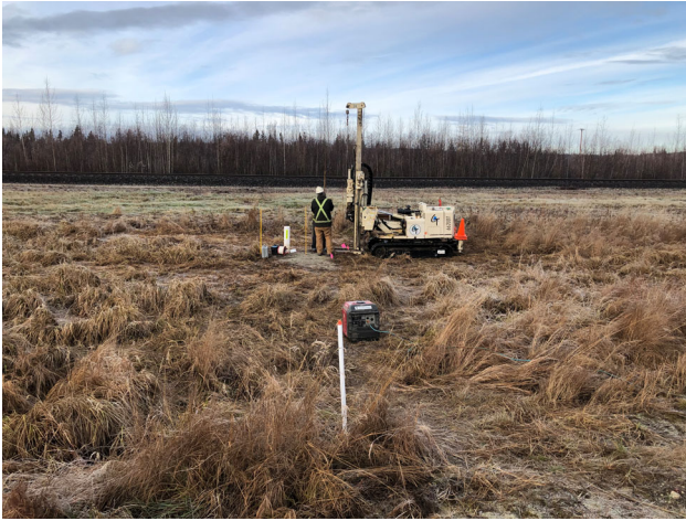
Photo 1: GeoTek advancing an injection well, October 29, 2019
