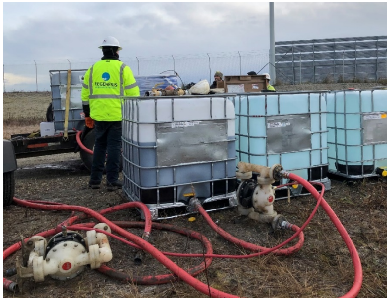
Exhibit 2-3: PlumeStop® and water containers at the injection site.
